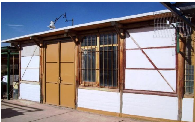
Fig. 9. Workshop with finished wattle and daub walls.
