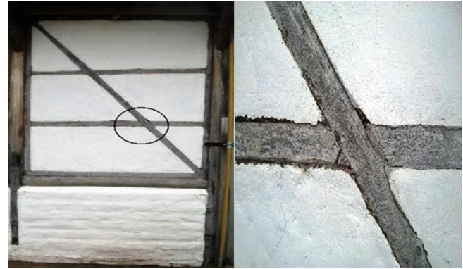
Fig. 14. Pathologies in joints on wattle and daub walls: a- Northern wall. b- Detail exterior joint.
