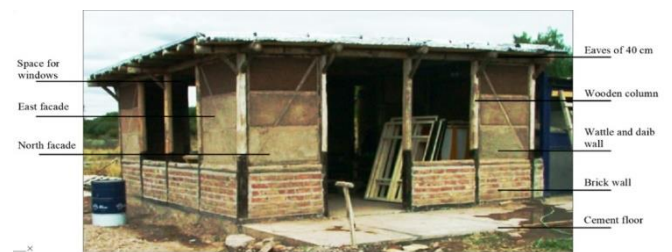
Fig. 11. Workshop construction stage.
