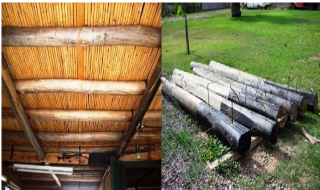
Fig. 8. a-Cane roof and b- Eucalyptus wood columns.
