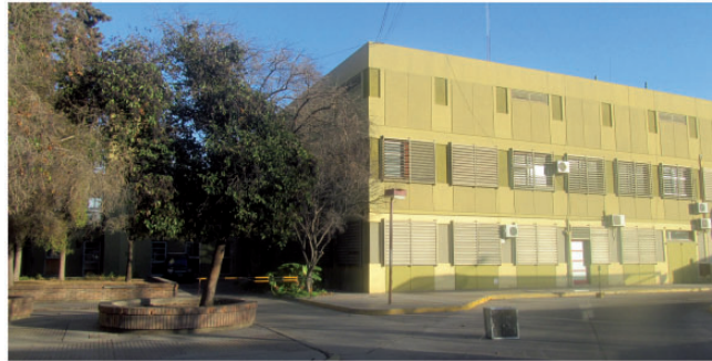
Figure 3. East façade of the area of analysis
