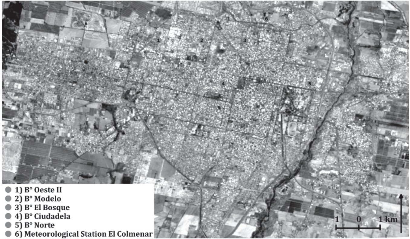
Fig. 1. Aerial photograph of the study area in San Miguel de Tucumán, northwestern Argentina.
