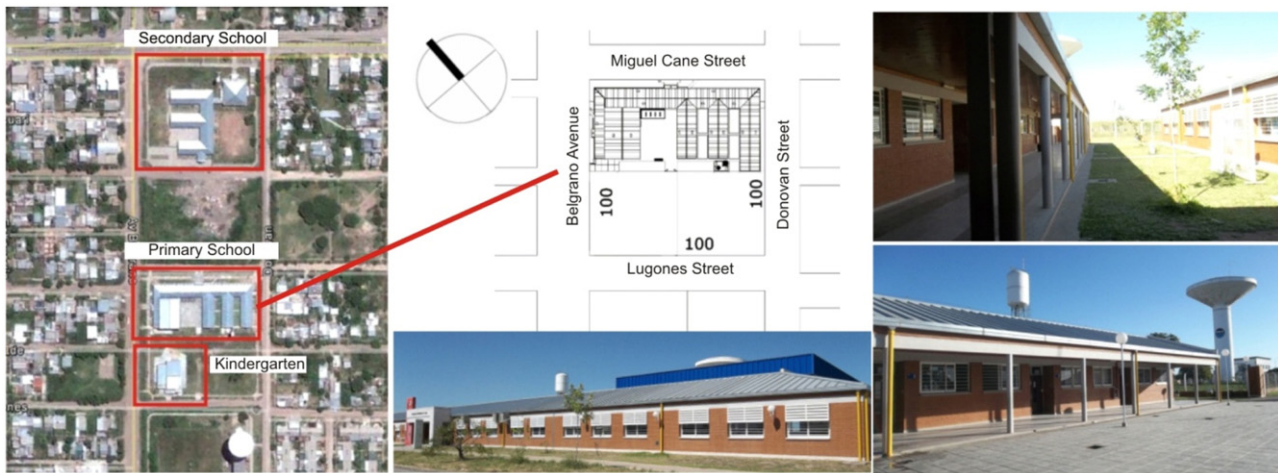
Fig. 1. Primary School Location and pictures of its highly exposed to direct solar radiation facades.
