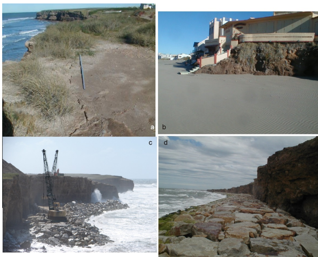
Figure 4 - Cliffs from Mar del Plata (38° S, see figure 1 for location). a) Fracture cracks on the top of the cliffs. b) Sea-side constructions are usually located attached to the cliffs composed of indurated siltstones. c) Rock revetments under construction. d) Armored structures are today protecting some cliffs.
