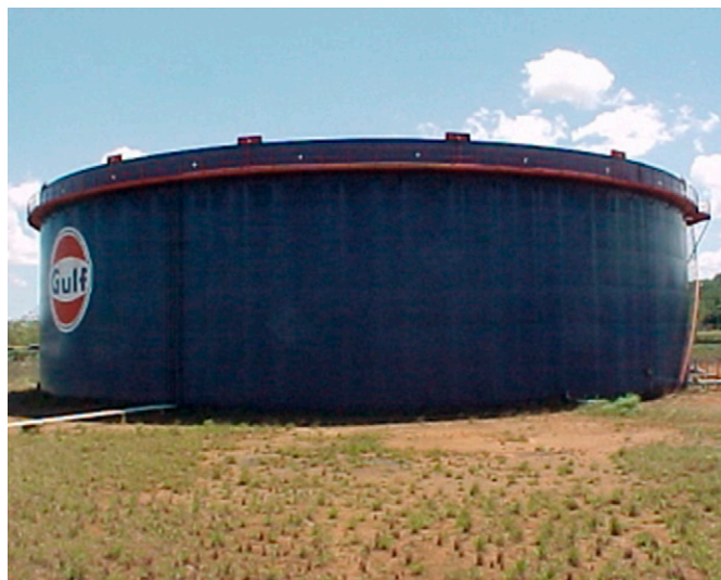
Fig. 1. Tank without external fixed roof located in the CAPECO Bayamon tank farm before the 2009 accident
