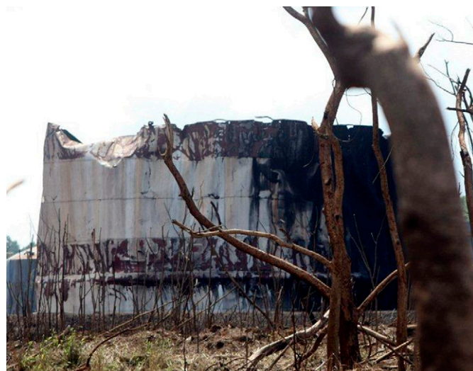
Fig. 3. Deformed configuration of a tank without external fixed roof after the Bayamon accident occurred in 2009 (with permission from GFR Media, LLC)
