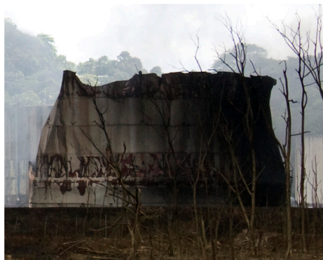
Fig. 4. Deformed configuration of a tank without external fixed roof after the Bayamon accident occurred in 2009
