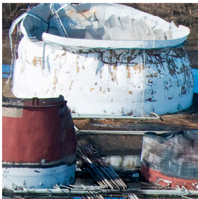
Fig. 6. Deformed configuration of a tank without external fixed roof after the Bayamon accident occurred in 2009
