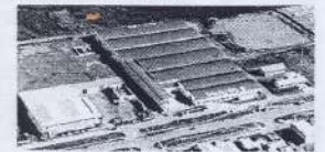
Fig. 42. Philips' facility today.
