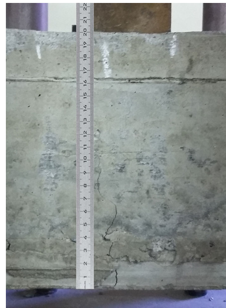
Fig. 13 Crack of Beam 02
