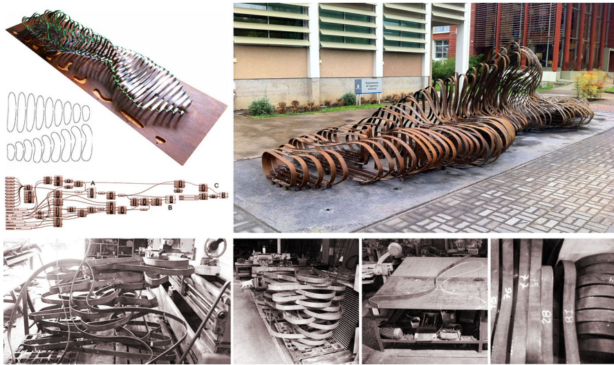
Fig. 9 BANCAPAR. Parametric installation under construction, Concepción, Chile
