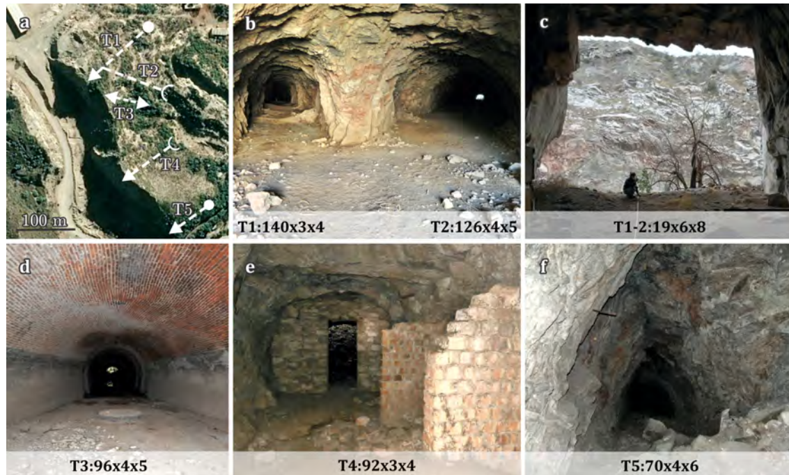
Figure 1. (a) Position of the tunnels (T) inside the old concrete factory. The ends of each tunnel are marked to denote whether they are open (arrowhead), partially obstructed (semicircle), or completely obstructed (full circle). (b,d–f) Each tunnel and their dimensions in metres (length, height, width). (c) Section of the tunnels that connects T1 and T2, and their dimensions.
